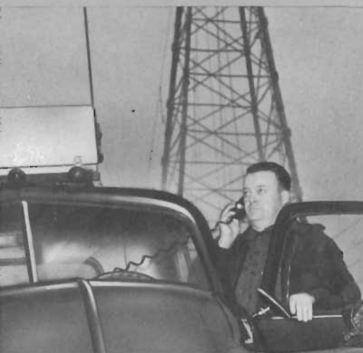
Remote Control—Unattended Stations
