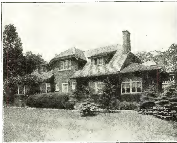
Fig. 1. Homes of this type lend themselves readily to the placement of radio outlets in each of the rooms with the receiver in a central location. The work may be done either while the house is in the course of construction, or else after the building has been completed
