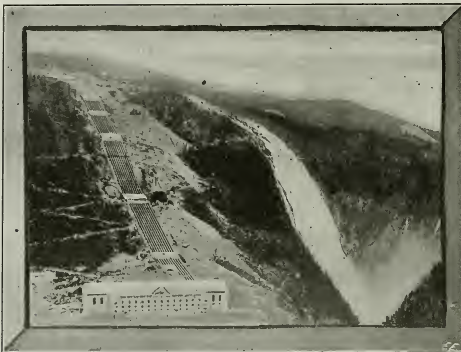
The Above View Shows the Gigantic Hydro-Electric Generating Station for the Fixation of Atmospheric Nitrogen at Rjukan, Norway. The Great Power of this Station can be Appreciated by Noting the Large Number of High-Pressure Water Pipes Leading Down to the Electric Generating Station, and Which By-Pass the Necessary Water From the Large Waterfall. The Station Is the Largest in the World and Develops 250,000 Horse-Power.
