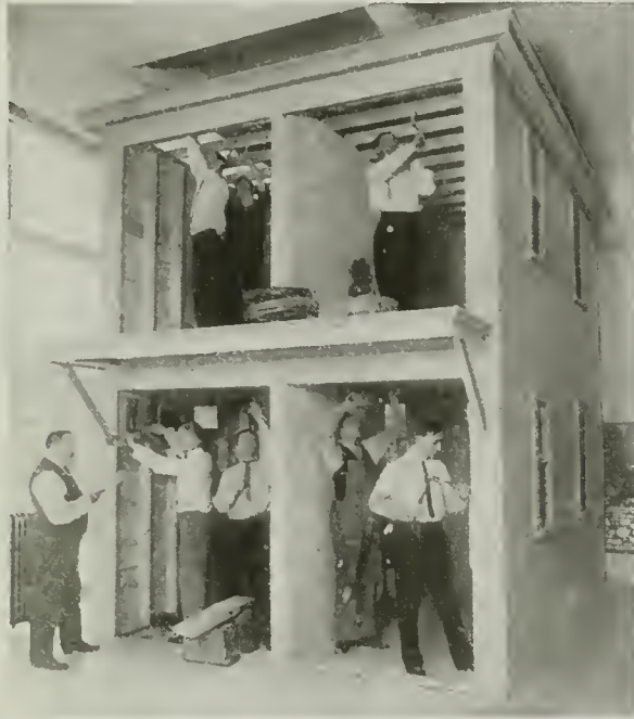
Students Completely Wiring Model House in School
