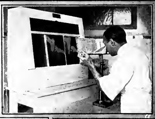
The "Radio-stereoscope" is the latest in French X-ray apparatus. By its means it now becomes possible to rapidly locate bullets or fractures—owing to the perspective of vision thus afforded. The X-ray plates are illuminated from behind, while the physician views them thru the special coordinating instrument shown. Fig. 3.
