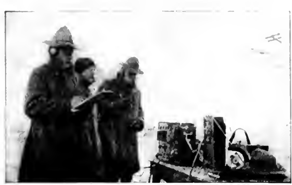
Ground Officers of the U. S. Army Talking to Airplanes in Flight by Means of Wireless Telephone. The Range of Such Communication Has Recently Been Increased to 150 Miles by Official Test.
