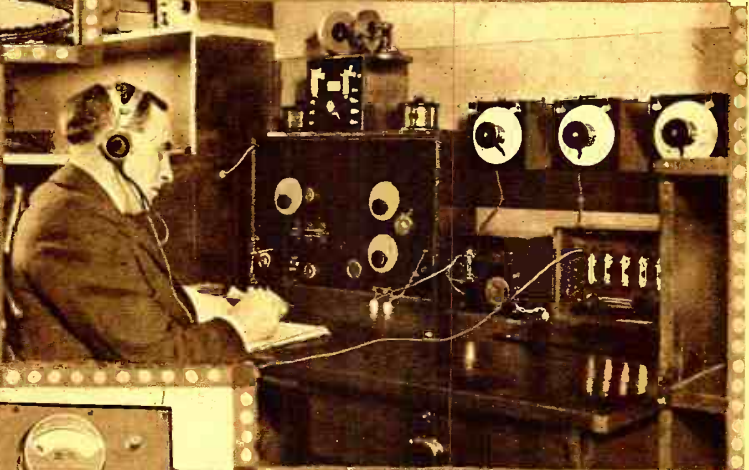
Below: View of the transmitting panel of CKAC, Canada's largest broadcasting station and the only one in the world that broadcasts in both French and English. It is operated by the French newspaper "La Presse." Instead of employing the usual motor-generator, the supply is obtained from the city A. C. current mains, being converted to D. C. by means of large rectifying tubes. The controls are such that only one operator is necessary. This station transmits on 430 meters.
