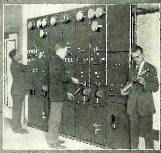
CONTROL PANEL OF WJZ. Every part of the complicated apparatus of the transmitting station is controlled from this one panel. The man on the right is holding one of the 10 kw. power tubes.
