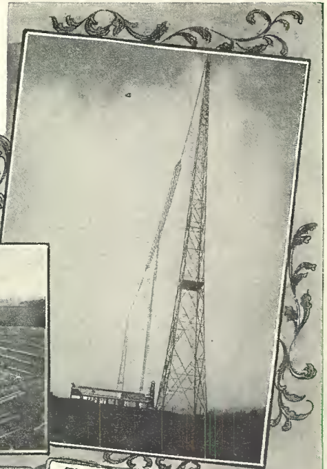
The building and aerial system at Langenberg. The towers are braced only by their own structure, and designed for minimum wind resistance. The cooling tower may be seen beside the lead-in.
