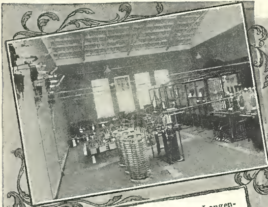
Interior of the transmitting room at Langenberg, showing the large inductances used, and the operating panel, wires from which operate the switches on the wall at the left.
