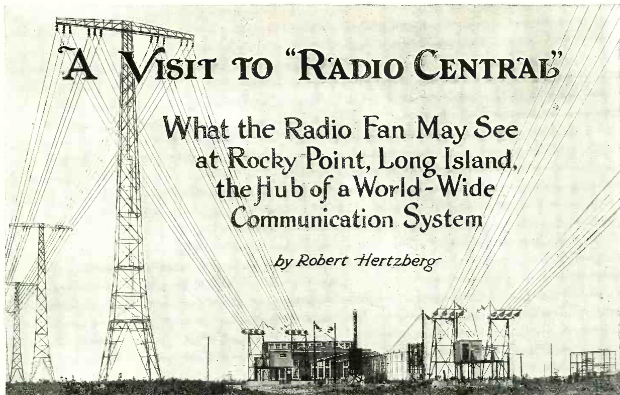
The scene above includes the main transmitter house at "Radio City", and the lead-ins from the two great aerials; the nearest towers of one aerial are seen at the left. They are 410 feet high.
