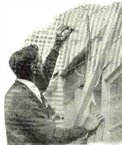
Norman McConnell, operating at Pylon No. 2, is shown at the left. At the right, Al H. Gyssler (W8BXB) is using a neon tube to find the nodal point on the antenna system at the headquarters station
