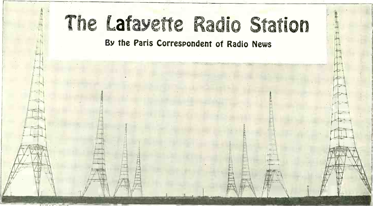
General View of the Lafayette Station Erected at Bordeaux, France. The Eight 835-Foot Towers Were Furnish and Erected by the American Navy. Note the Building in the Background.
