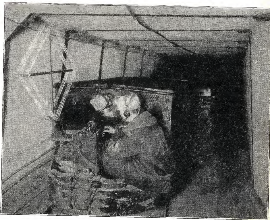
An experimental loop receiver mounted on a storage battery locomotive. This and similar apparatus is being used to study the attenuation of waves in penetrating the earth.
