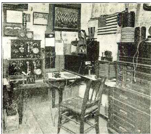
Photograph of Mr. Giblin's Original Amateur Station Located at Pawtucket, R. I., Where the First Honeycomb Coils Were Tested Under Actual Receiving Conditions, the Event Taking Place Several Years Ago. Note Several of These Coils on Top of Cabinet in Right Hand Side of Picture.
