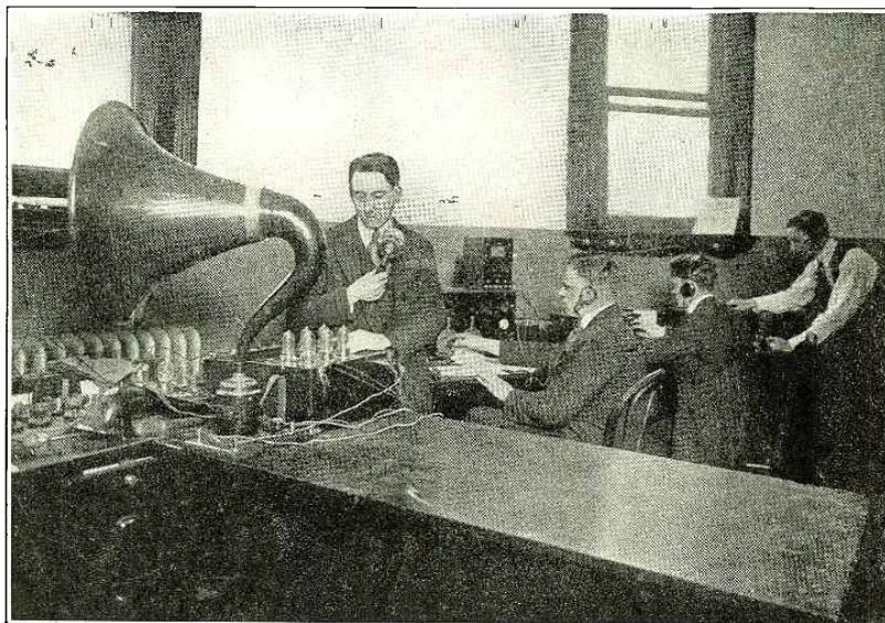
Interior of the Radio Receiving Station in the Tower of the Times Building, New York City. Note the Sound Amplifying Instruments to the Left of the Picture Which Were Used to Receive Secretary Daniel's Voice from the U. S. S. Pennsylvania to the Heart of the City.
