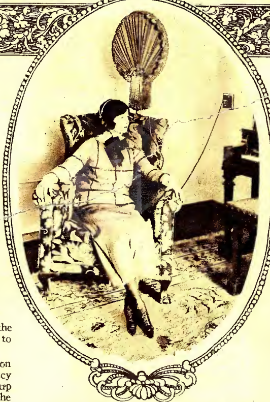
The Ritz Apartment In Newark, N. J., Is One of the First to Give Tenants Complete Radio Service. A Sensitive Radio Receiver Picks Up the Concerts, Which Are Then Magnified By a Power Amplifier and Carried By Wire Direct to Each Individual Apartment. A Plugging Arrangement in the Walls Makes It Possible For the Tenants to Listen In At Will. The Photo In the Upper Right-Hand Corner Is That of the Receiving Set Installed on the Roof of the Ritz Apartment House.
