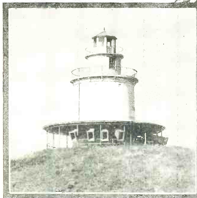
The odd structure above serves, not only as a lighthouse, but also as a community radio loud speaker. It is located at Dartmouth, Mass., where the Round Hills Radio Corporation maintains station WMAF. Around this battery of huge speakers the whole population of the town may gather on pleasant evenings to hear programs reproduced with a volume that fills all outdoors.
