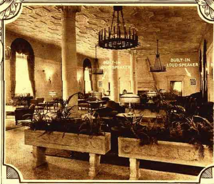
Above, a view of the foyer in the recently completed Pennsylvania Hotel in Philadelphia, shows one of the built-in loud speakers, many of which are situated at different parts of the hotel. These are all connected together and are operated from the same source.
