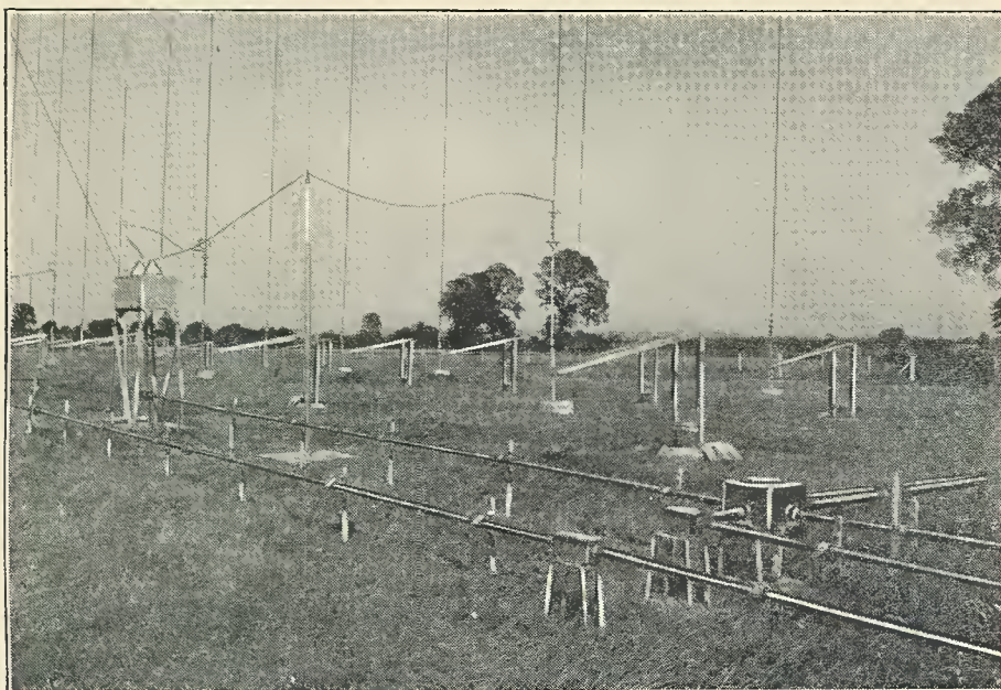
At the lower right are shown the feeder lines for the antenna, with a junction box; on the left an antenna coupling box, and the antenna balance weight system in the background.
