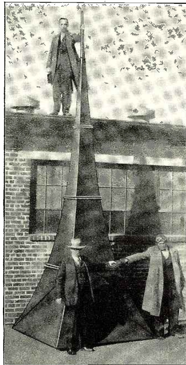
Mr. Dey is standing directly in front of his 20-foot exponential horn. Its size may be gauged by comparison with its surroundings. (It is not recommended for use in a portable set).
