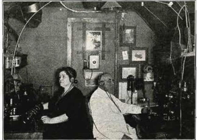
The Radio Room at 9XAG. On the Right May Be Seen the Radiofone Set and on the Left the Motor Generator.
