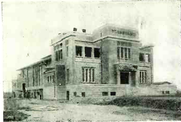
Above is an illustration of the recently-completed administration building of the station at Monte Grande, near Buenos Aires, which links the Argentine Republic directly with Europe. Below, a glimpse of the transformer room.
