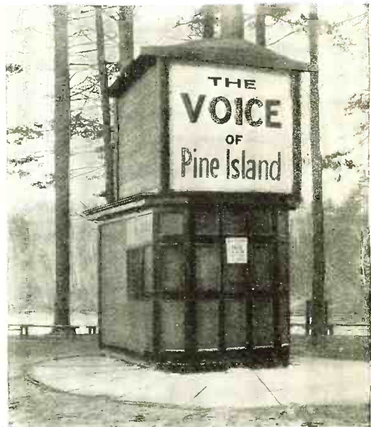
Large exponential horn used at Pine Island Park, Manchester, N. H., to provide public concerts from phonograph records
