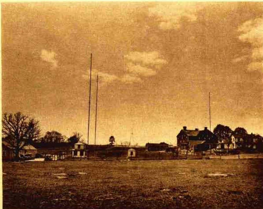
The radio shack and the two immense 100-foot towers which support the aerial of station 8BRC. Another aerial atop Mr. Myers' house is employed for broadcast reception.
