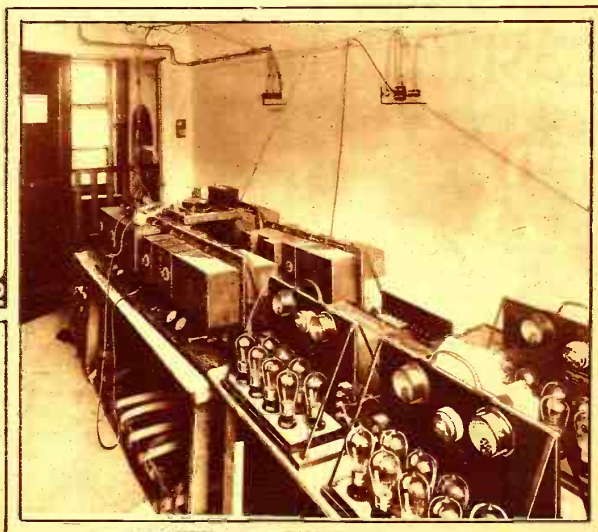
At the left, one of the loud-speaker units used at Hendon. The phone used for communication from the ground to the airplanes was connected with a system of amplifiers, so that all orders were audible to the crowd, who could watch the movements of the aircraft in response to them. At the right below is shown the battery of amplifier which furnished current to the loud-speaker units about the field.
