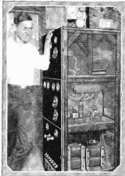
The short-wave transmitter of 2XAL is small and simple, but carries farther than high-power stations on long waves.
