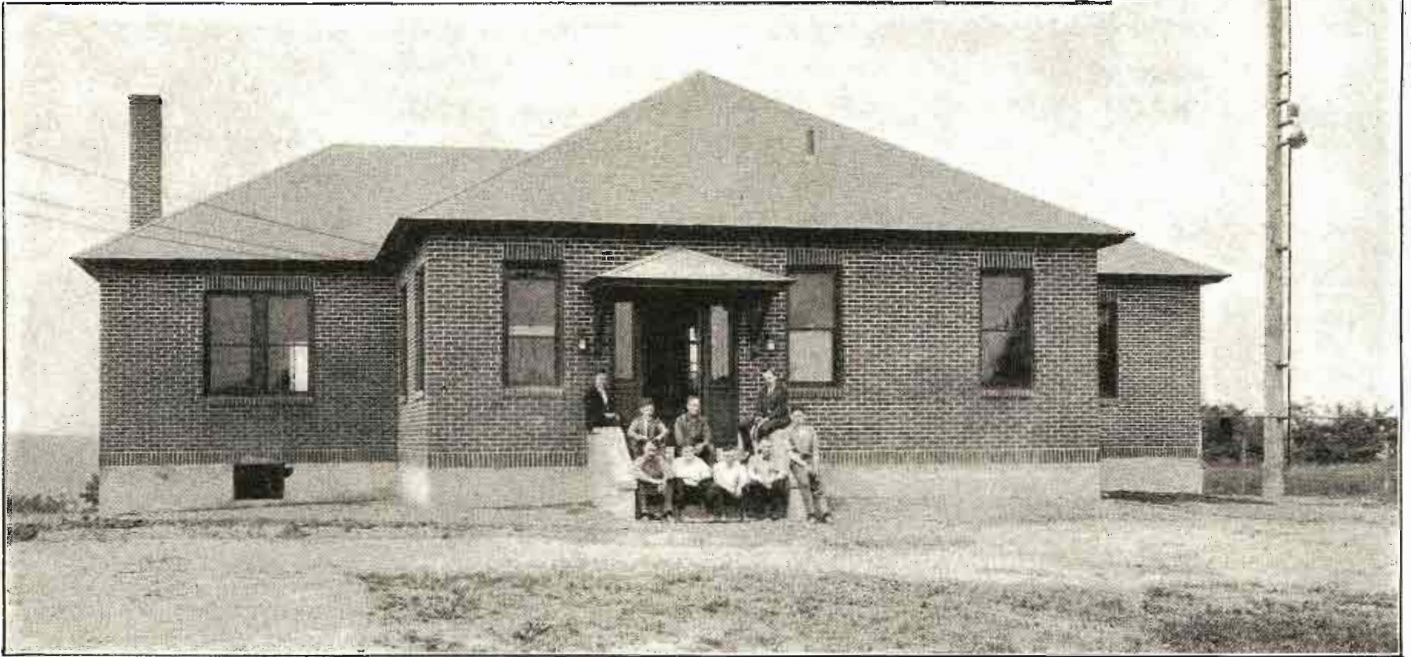
The new Westinghouse experimental building in which is located KDKA's short wave transmitting station. The unique vertical antenna, consisting of about 50 feet of copper tubing, is seen at the right.
