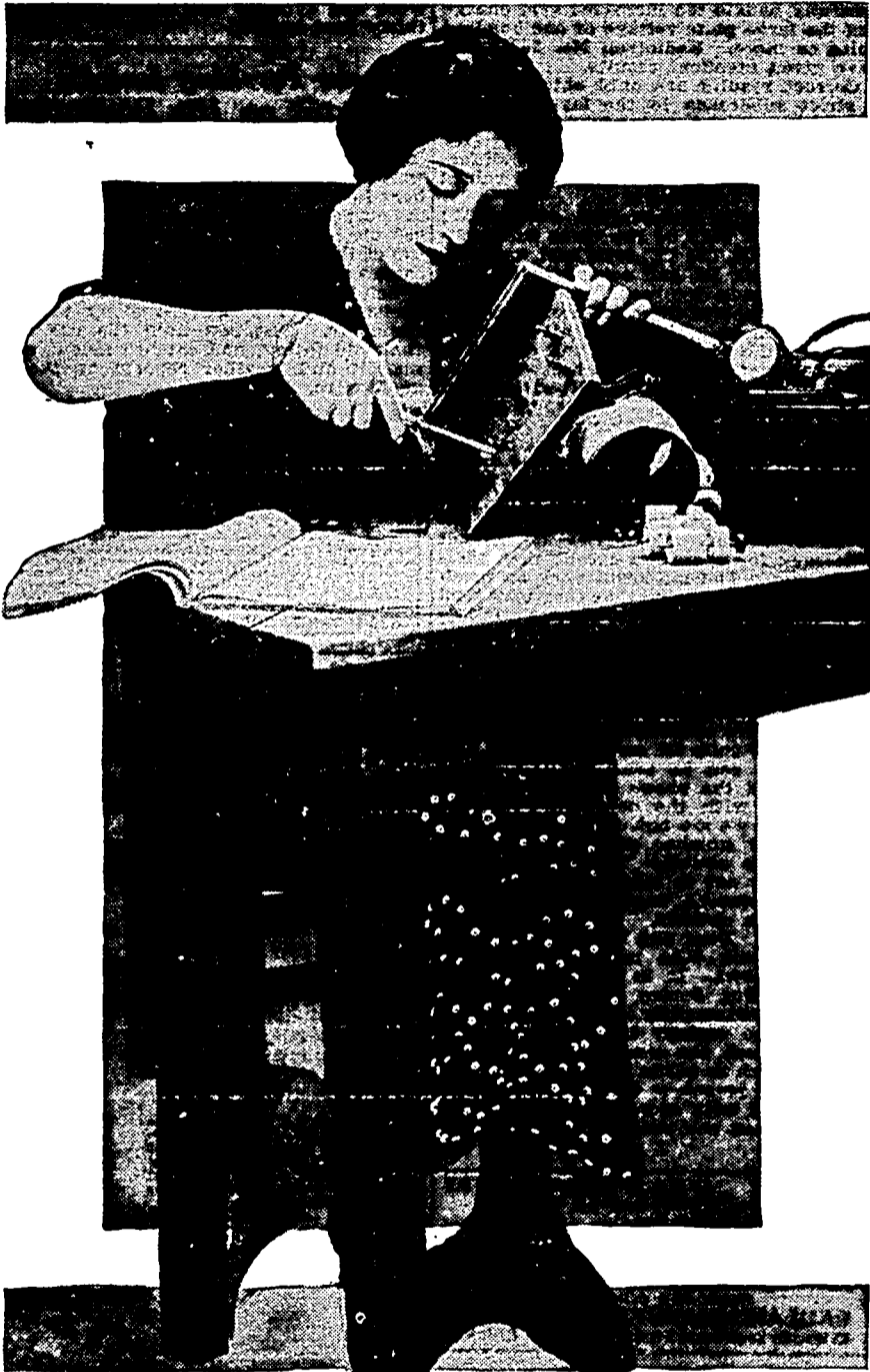
Radio has such a strong grip on the nation that many of the girls, not satisfied with mere listening in on brother's or the neighbor's outfit, have undertaken to build their own. And the ladies are clever; our friend in the photograph has used a salt box upon which to wind the coil Photo by Hoover Art Studio
