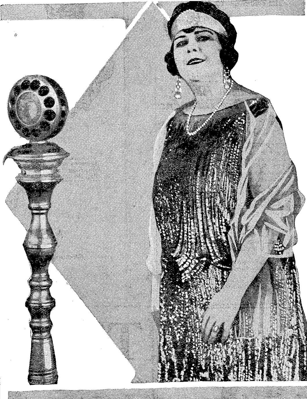
Perfect synchronization of sound and motion so as to supply the missing link of speech between the screen actor and the movie fan was promised not long ago by Dr. Lee De Forest as a development of the near future and is now ready for demonstration before the public. Here is seen Mrs. De Forest singing before the microphone while her motions are recorded by the movie camera K. & H. Photo
