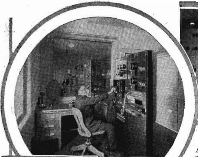
Control room, showing operator sitting at desk. He has a clear view of the transmitting panel through a plate glass partition.
