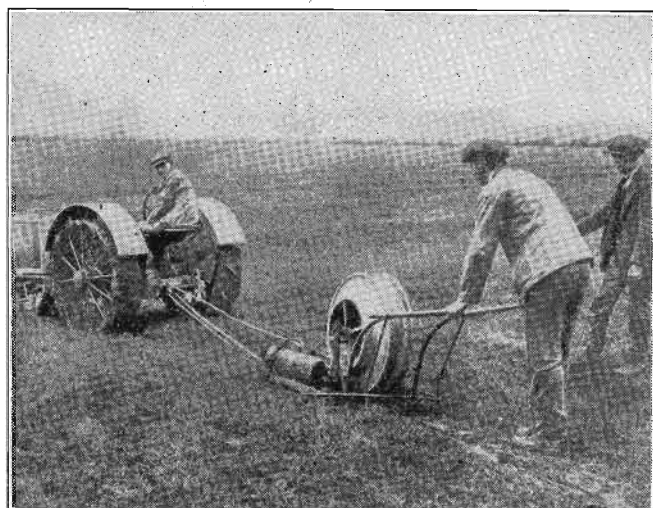
W EAF with its 50,000 watts is small potatoes compared with the new British Post Office station at Rugby, which generates 540,000 watts. Picture shows special plow that turns up a furrow just wide enough to take the wire from the drum, mounted behind.
