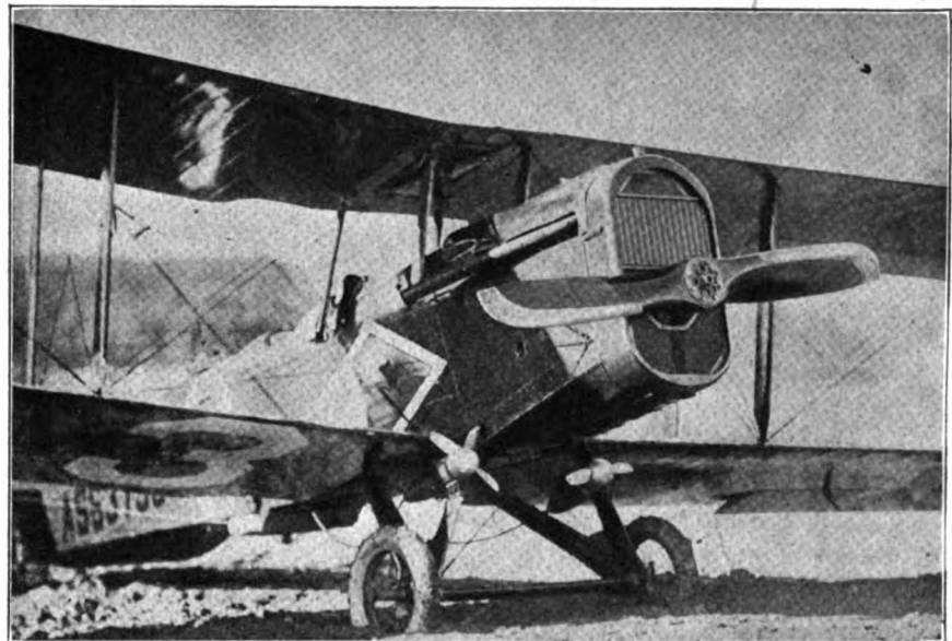
Double installation of fan-driven generators on 'plane. This double installation is made on 'planes making long patrols and trips, where communication is imperative, especially when the 'plane is used for fire patrol work.
