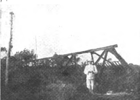
The Fallen Wireless Tower at Duala.
