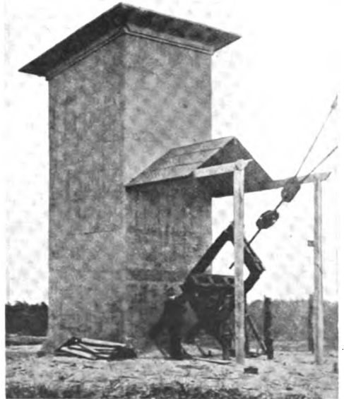
One of the Concrete Anchors to hold the Wireless Towers.
