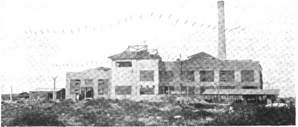
Power House (note Insulators on 32 Aerial Wires).
