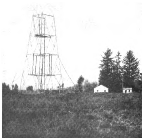
Astoria Station—Two forward Towers under construction.
