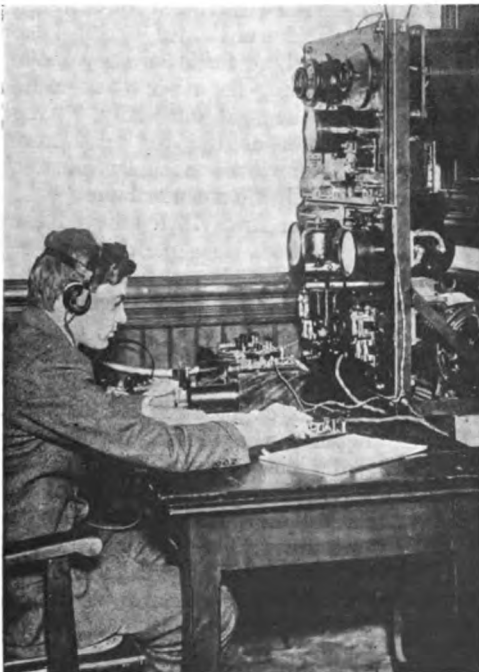
Wireless Installation at New York Fire Station.
