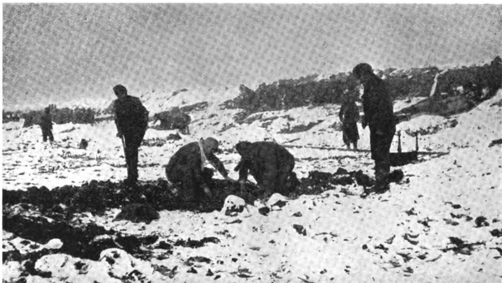
The difficulties of Erection of Wireless Masts during Winter Campaigning.
